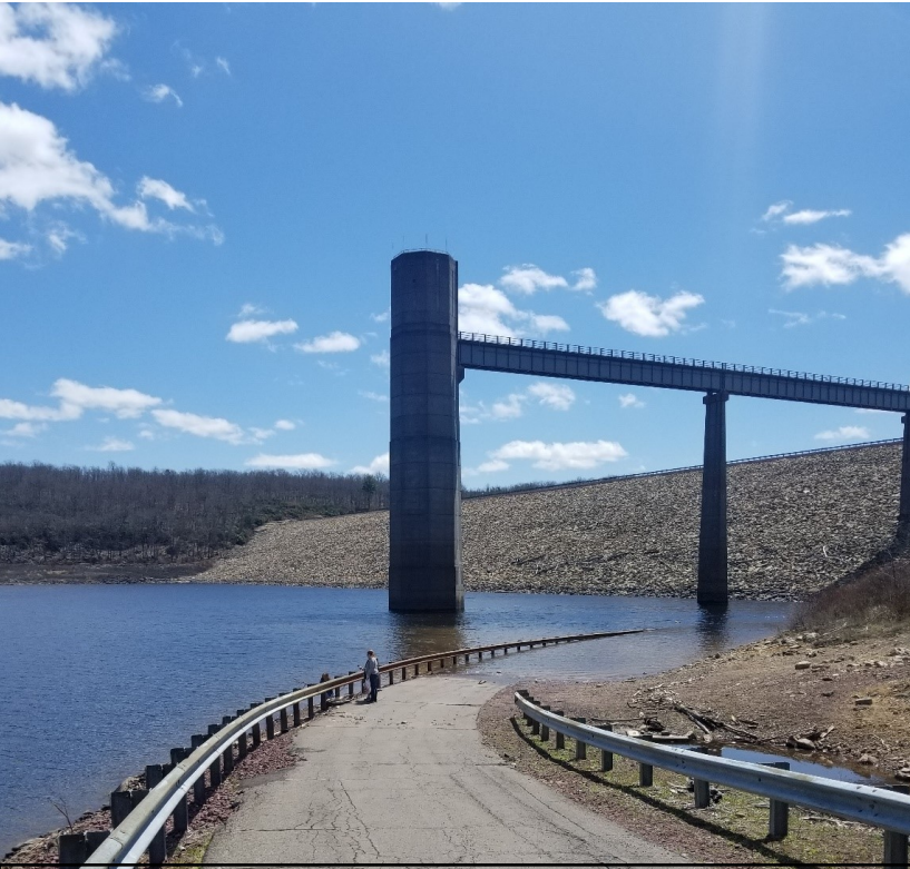
The flow control tower at Francis E Walter Dam
